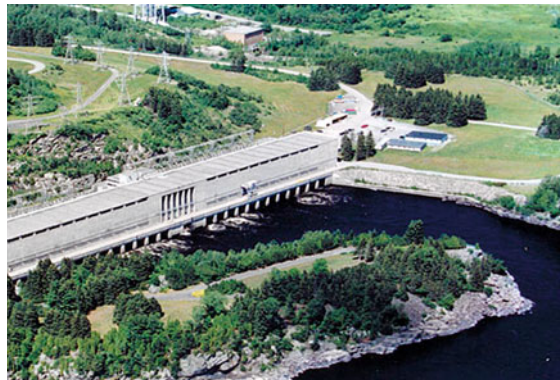
Shipshaw HPP (courtesy of Alcan Canada)
